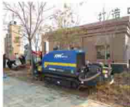
银川施工现场 Job site in Yinchuan
